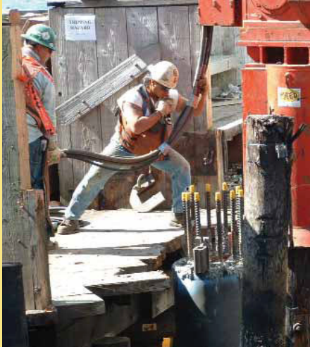
Pile buck talks to crane operator during removal of old piling.
