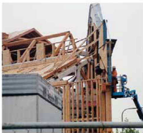
Carpenters Work on Aquarium Façade and Entry
