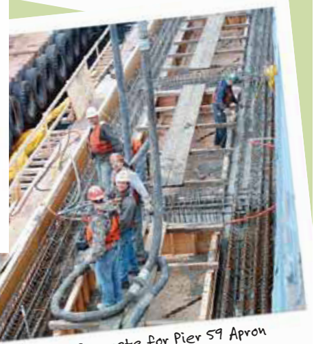
Laying out Rebar for Pier 59 Concrete Apron
